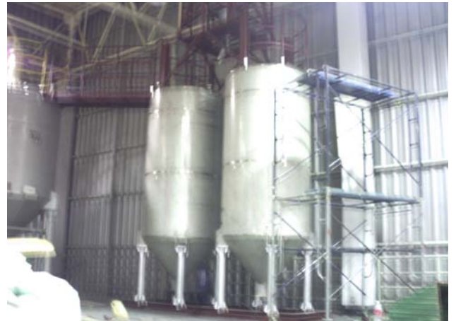
Storage Tank size,6.0 m 3 ,SUS 304
